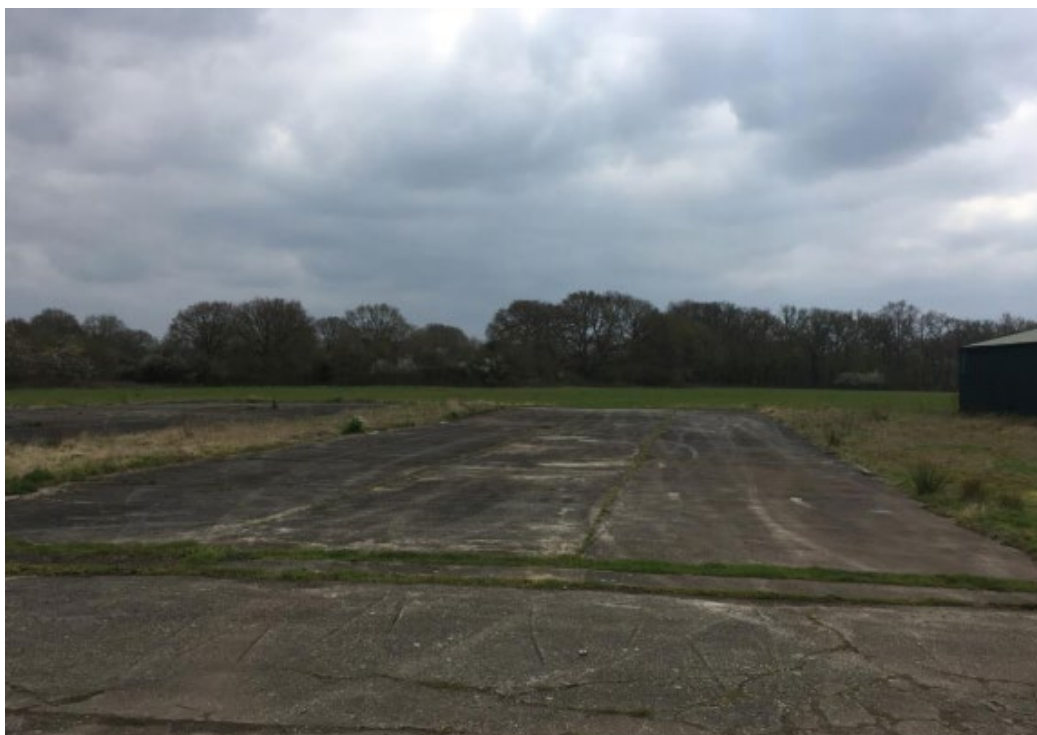
Figure 8: Existing concrete slabs
