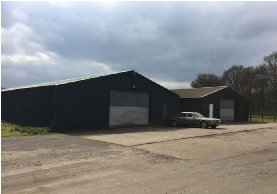
Figure 6: Existing Buildings (Enclosed Barns A and B)
