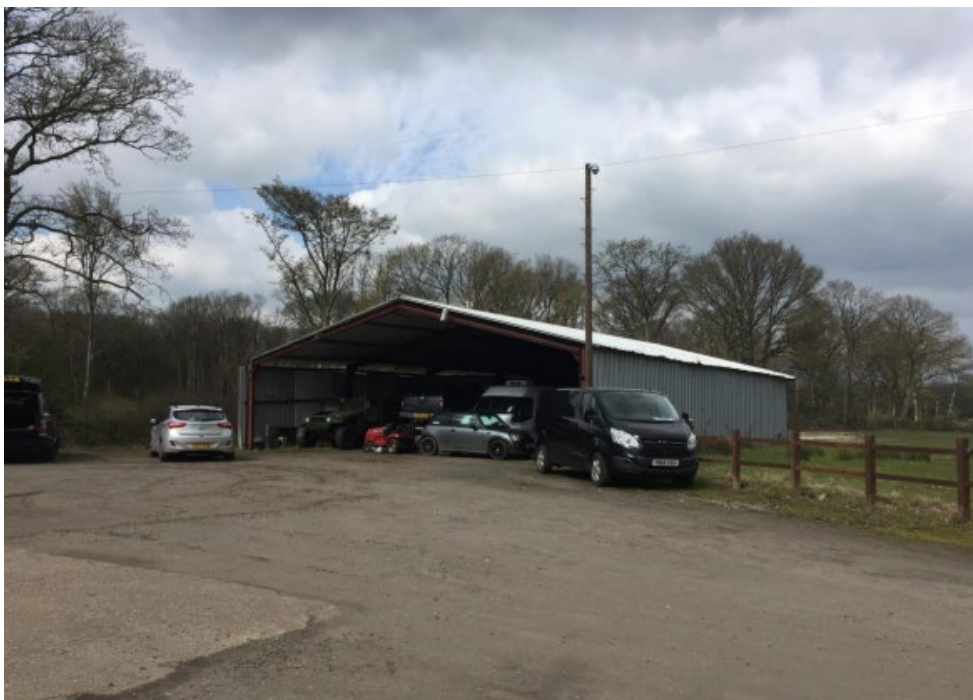
Figure 7: Existing Building (Open Fronted Barn C)
